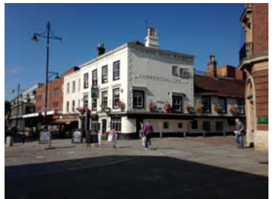
The crossing point of South Street/North Street and Market Place in the centre of the Conservation Area
